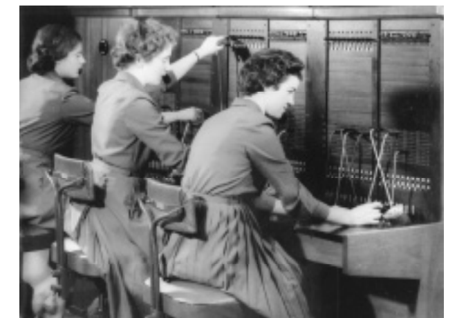
ICI House, East Melbourne, Telephone switchboard, 1958. Wolfgang Sievers. National Library of Australia
